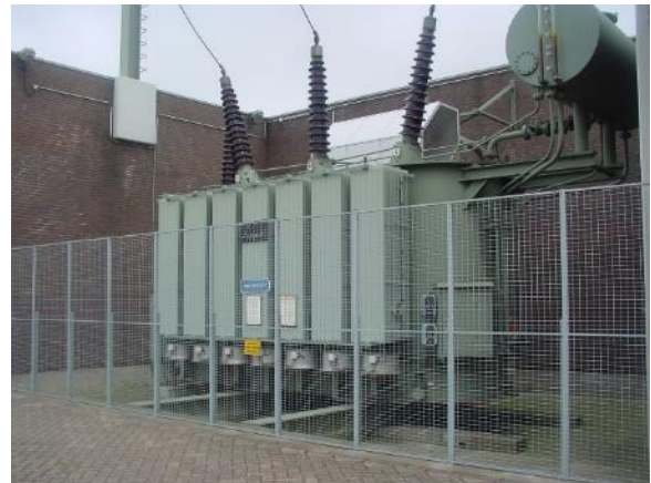
HS/MS-transformator
