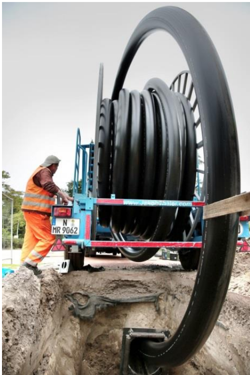
Close-Fit lining, Breda 2015
